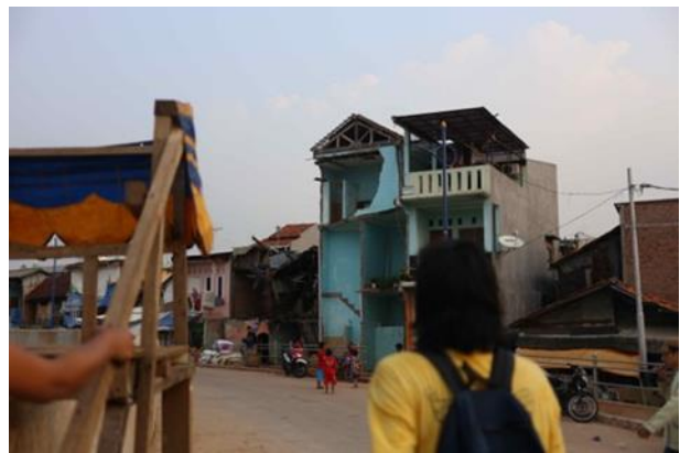
A house broken by the river bank construction in the Pulo village.
