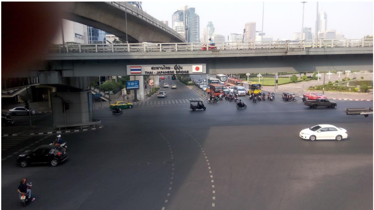
The Thai - Japanese bridge in Bangkok
