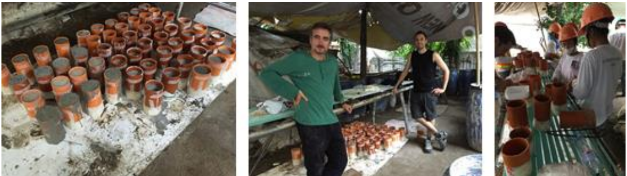
Picture 6. Construction of traditional mortar cylinder in Malate church, Manila
